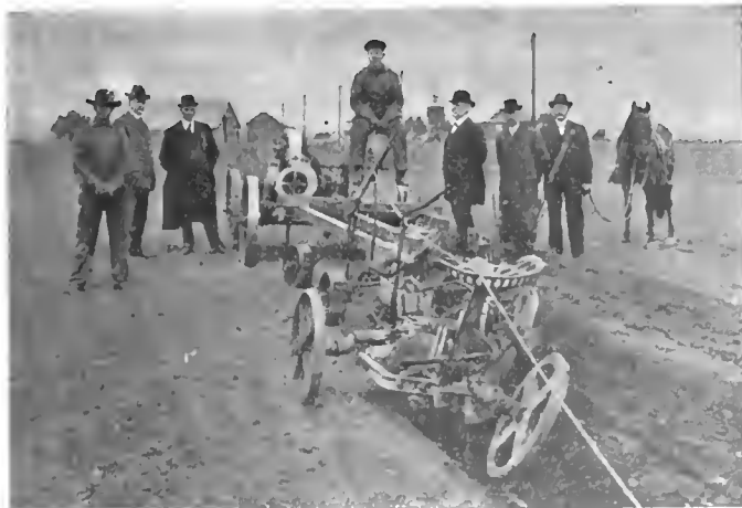
REAR VIEW SHOWING CABLE AND MACHINERY IN TOW.
